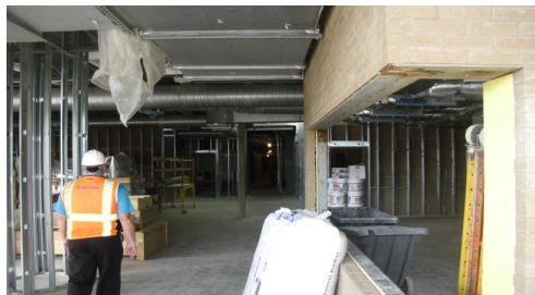
View of Visitor Entrance to the New Lab
