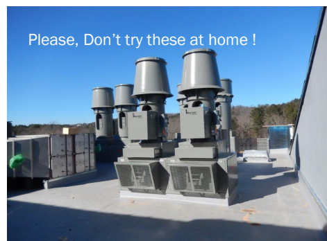
Huge Air Handling Systems on New Lab Roof
